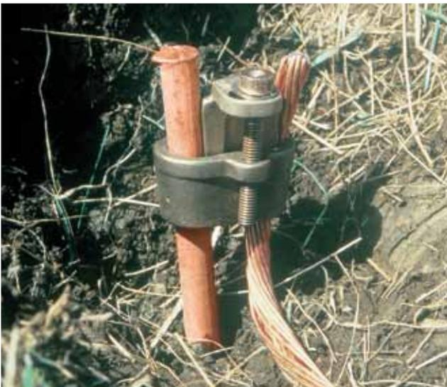
DSA Copperweld® wire and strand have the high current-carrying capacity characteristics in short-time durations, high strength properties and corrosion resistance to effectively and economically meet IEEE recommendations. These advantages are particularly evident when compared to a low-strength material such as solid copper. Solid copper conductors must be upsized in many installations to meet the mechanical demands within a system design.
